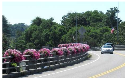
The Hooksett Memorial Bridge in August
