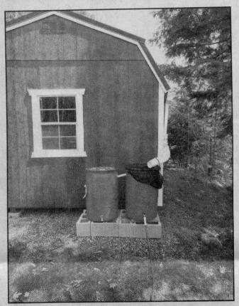
the downspout and \$12 for fittings. Scrap hose was used. The 55-gallon barrel was flipped on its side. The downspout was cut to put in the diverter. Piece by piece, the project took about four hours to complete.
